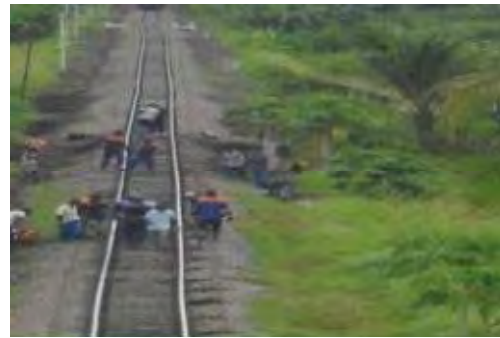
railroad employee was repairing the damaged railway
