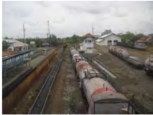
boiler fuel transporters
