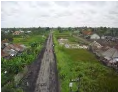
Situation around railway at Keramasan
