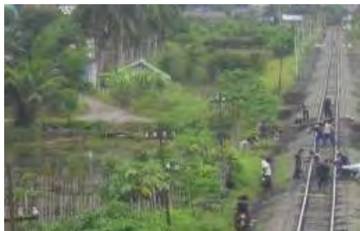
railroad employee was repairing the damaged railway
