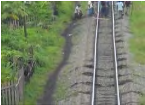
railroad employee was repairing the damaged railway
