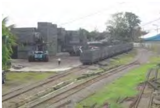
Situation at coal stockpile
