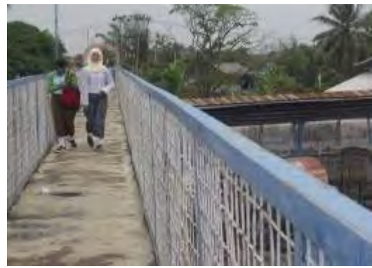
Accrossing Bridge in the Kertapati Station
