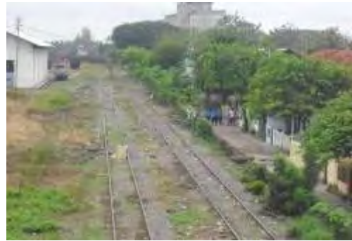
Situation near the railway line
