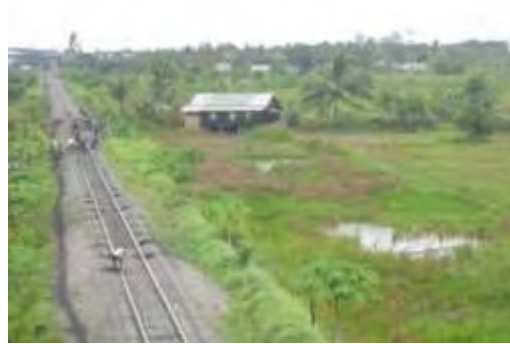
railroad employee was repairing the damaged railway
