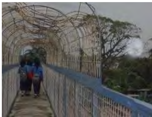
At the bridge in Kertapati Station
