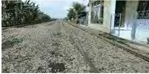
PC Sleeper is hidden by the ballast. (Simpang Station toward Kertapati)
