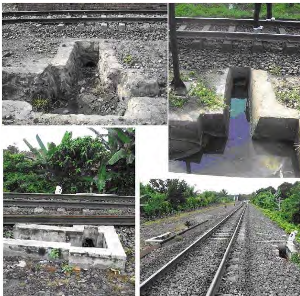
[Pic. 4-1-5] Present Condition of Lateral Drainages and Small Scale Culverts
