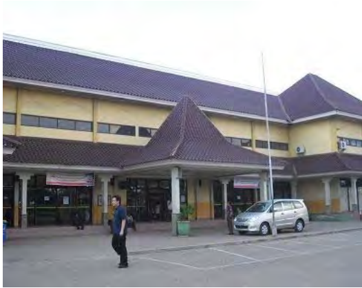
Kertapati station in renovation
