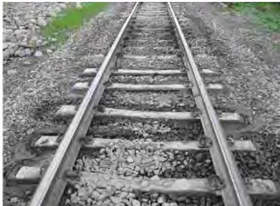
[Pic. 4-1-2] Mud Pumping on Tracks
