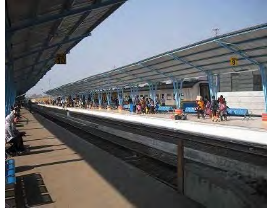
Its newly constructed platforms
