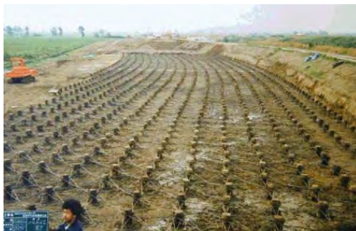
[Fig. 5-1-3] Overview Diagram of Method of Pile-Net
