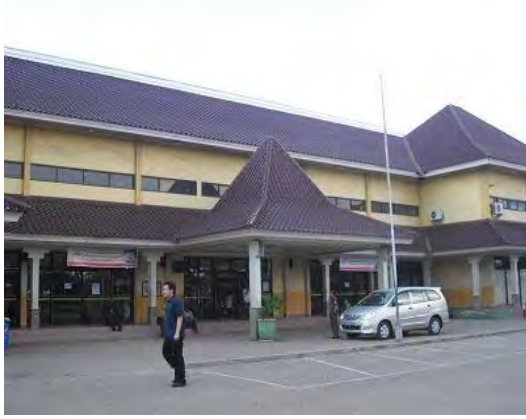
Kertapati station in renovation
