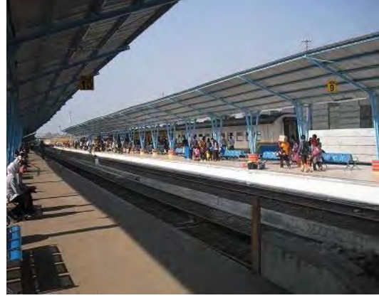
Its newly constructed platforms
