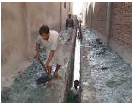
Figure 2-2 Channel Cleaning of Narrow Road
