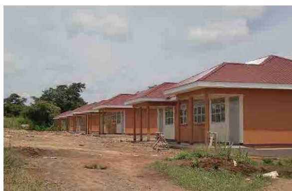
Figure 2.1.3 Amuru Staff House
