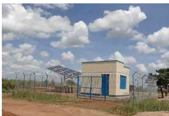
Figure 2.1.5 Pabbo Water Pump Facility
