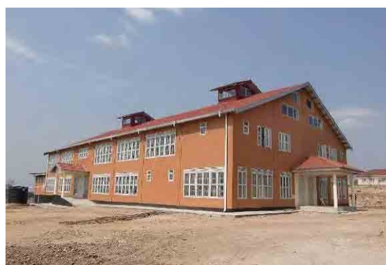
Figure 2.1.1 Amuru Multi Purpose Hall
