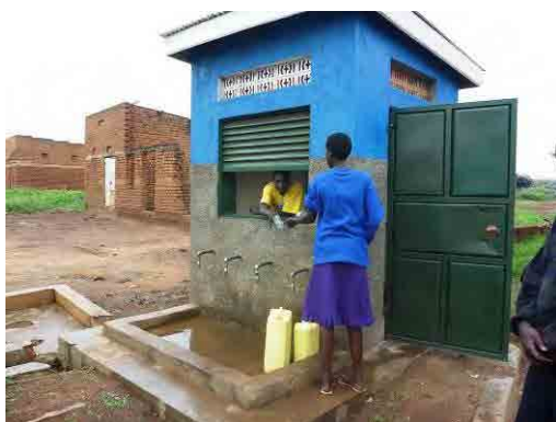
Figure 2.2.11 Water Kiosk in Lamwo District
