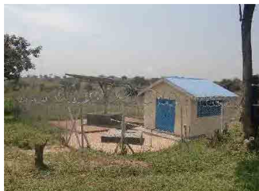
Figure 2.1.18 Water Supply Facility in Amuru District
