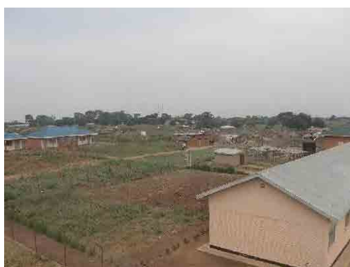
Figure 2.1.14 Garden surround the Facilities (4) Pabbo Sub-county: Staff quarters (Lot 4)
