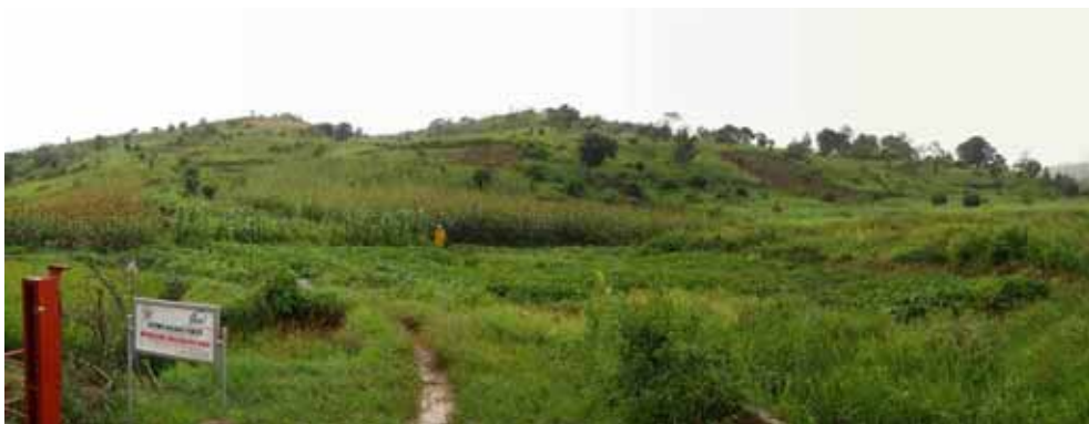
Dam Axis – Right Bank View
