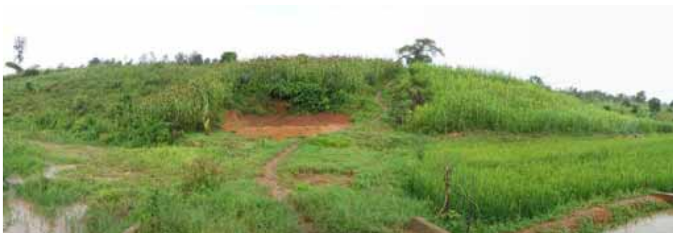
Dam Axis – Left Bank View
