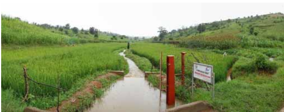
Dam Axis – Downstream View
