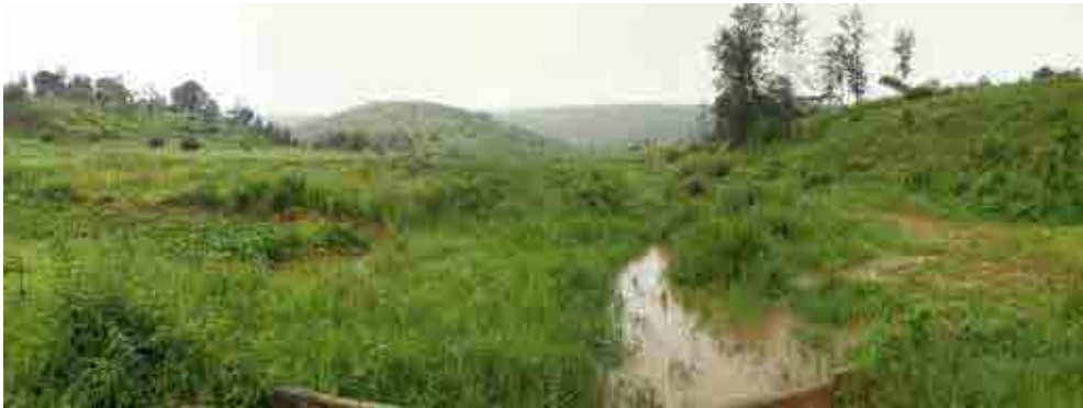
Dam Axis – Upstream View
