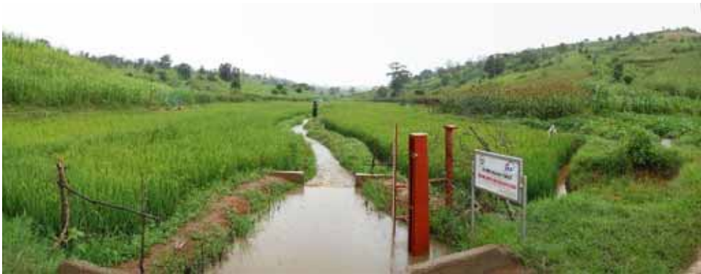
Dam Axis – Downstream View
