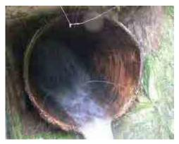
600mm steel pipe, corroded a little
