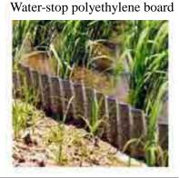
reduce the leakage through the ridge's foundation by the effect of penetrated walls. As the wall materials, there are many kinds, but the water-stop polyethylene board popular in Japanese market shall be suitable considering the durability and the economical conditions, i.e. high price of wood in Rwanda.
