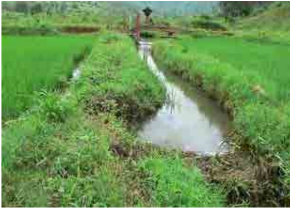
Downstream 50m, dam up and in-let mouth
