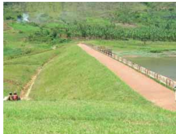
Protection work by grass on the downstream slope
