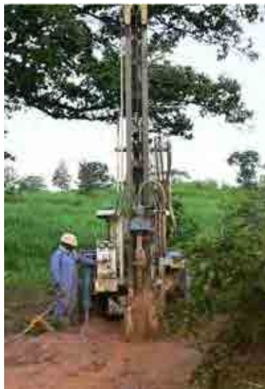
Status of test hole drilling
