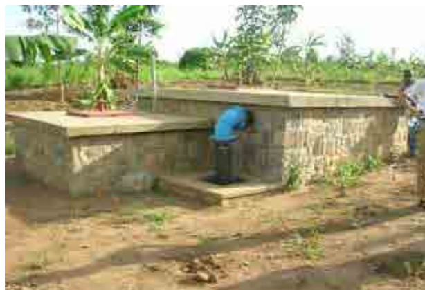
Tank placed on the upper edge
