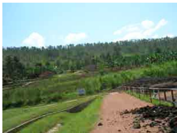
Dam ( Dam crest ~ right bank side )
