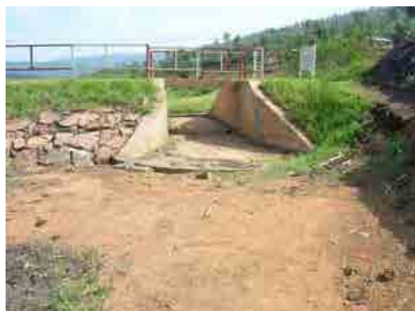
Spillway mouth ( spill out in April and November )
