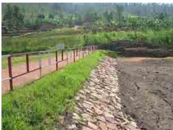
Riprap on upstream slope
