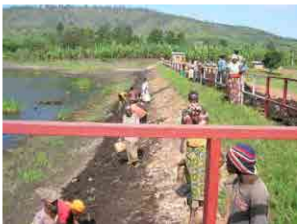
Dam ( Dam crest ~ left bank side )
