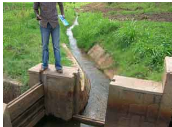
Division work( main canal on the right side )
