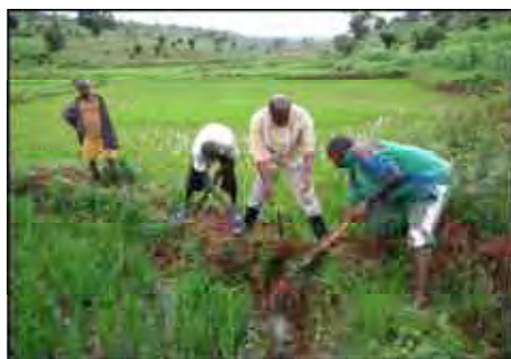
Picture-1.Repairing of the bund
