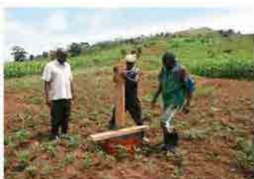
Setting of the buffering pond
