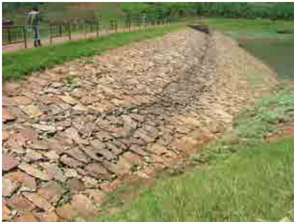
Riprap on the upstream slope
