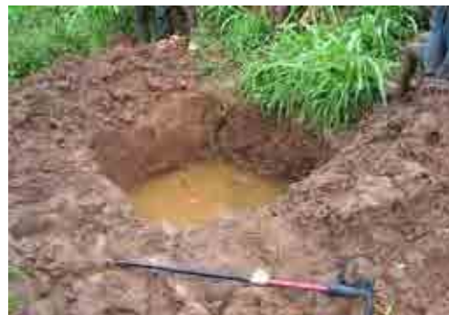
15 Water table in Test Pit-2
