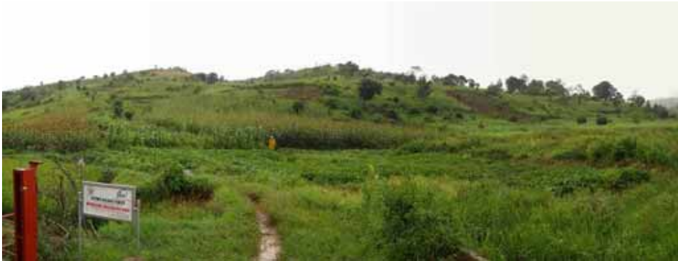
Dam Axis – Right Bank View
