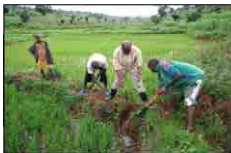
Repairing of the bund
