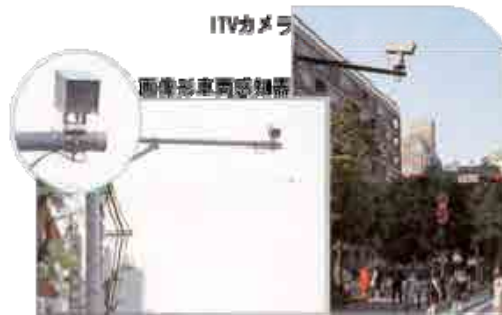
Figure 3.8.36 ITV Camera & Vehicle Detector
