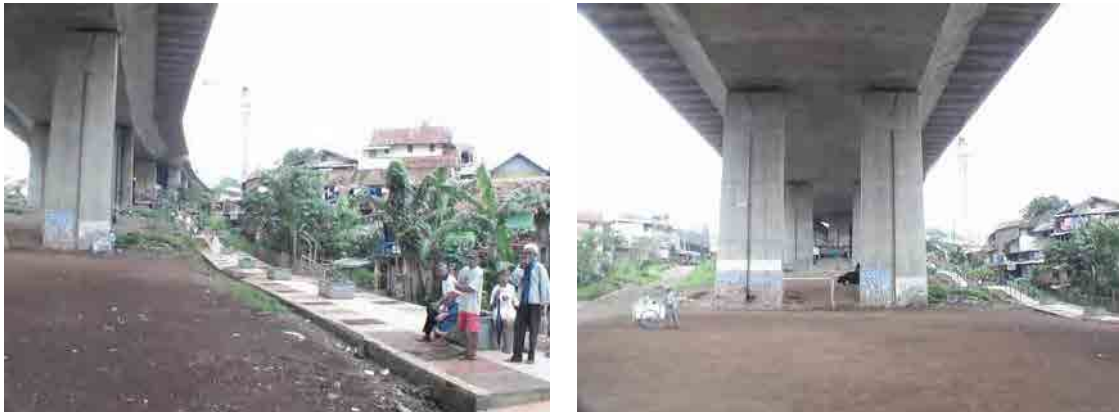
Photograph 3.7.5 Present Condition under Pasupati Bridge
