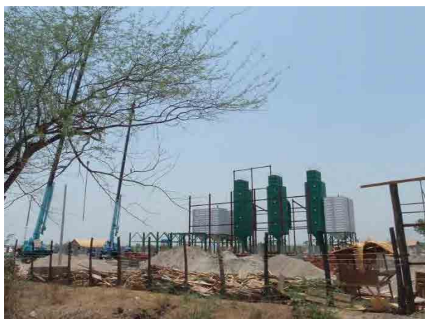
Post-harvest Facilities of Rice Specialized Company Complex under construction for drying: 300 tons /d, rice milling: 250 tons/d, seed cleaning: 4 tons/d, and storage: 15,000 tons. They plan to operate it, by purchasing rice from contracted farmers. [Minbu, Magway Division]
