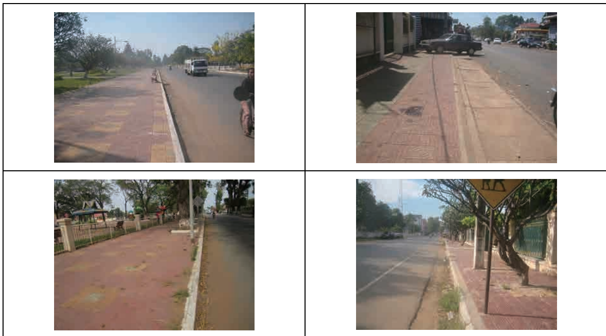
Photo 1 Existing Sidewalk Pavement in Kampong Chhnang
