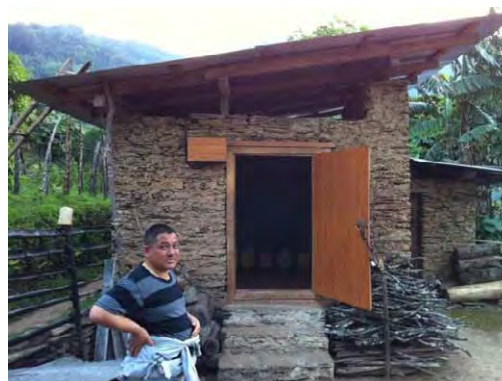
Improved storage for maize storage constructed by NPHC (Zhemgang)
