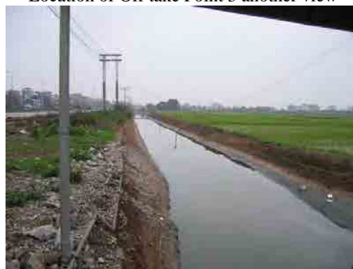
At Off take Point 4 pipelines will have to cross railways and drain through trenchless method
