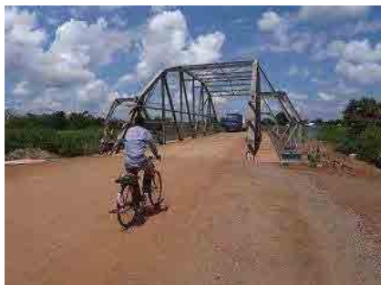
Newly Constructed Bridge across Border by USAID
