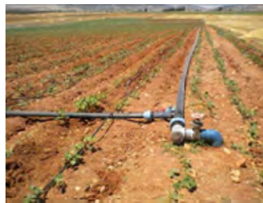
Hydrant (front right) and Drip irrigation system: distribution pipe and drip tube (GR)
