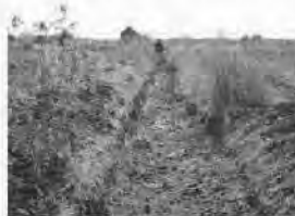
Canal in Middle Shabelle before rehabilitation
