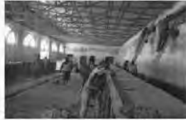
Rehabilitation of Fish Market in Hamarwoyno District, Benaadir Region
