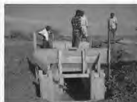
Culvert construction in Afgoye District, Lower Shabelle
