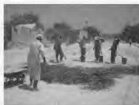
Road rehabilitation in Hamarjajab District, Benadir
