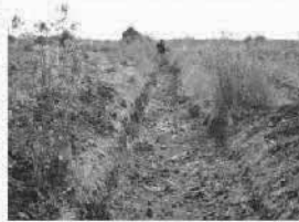
Canal in Middle Shabelle before rehabilitation
