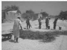
Road rehabilitation in Hamarjajab D district / Benadir
