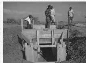
Culvert construction in Aigoye District, Lower Shabelle
