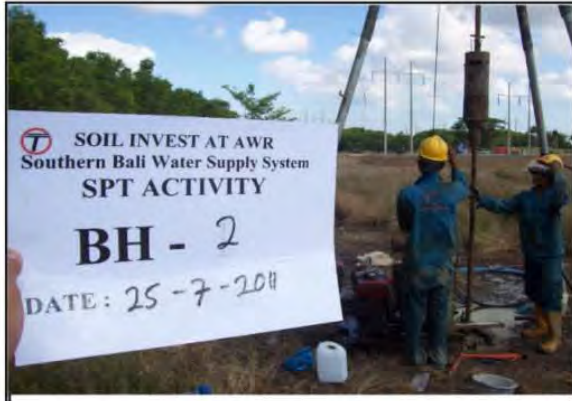
DRILLING AT BH-2
