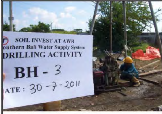
DRILLING AT BH-3
