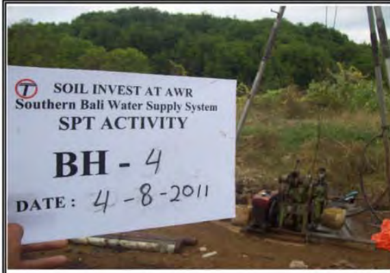
DRILLING AT BH-4
