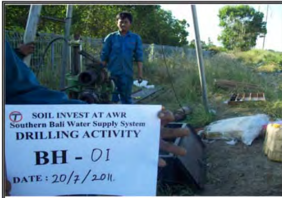
DRILLING AT BH-1
