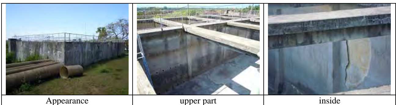
Figure 8.5.3 Present Condition of the Existing Reservoir
