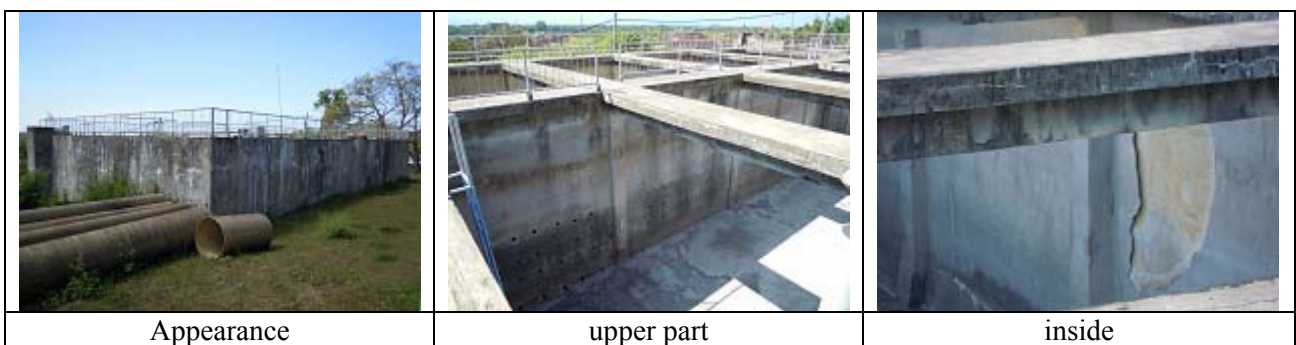
Figure 8.5.3 Present Condition of the Existing Reservoir
