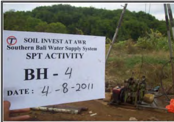
DRILLING AT BH-4
