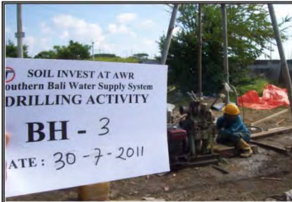
DRILLING AT BH-3
