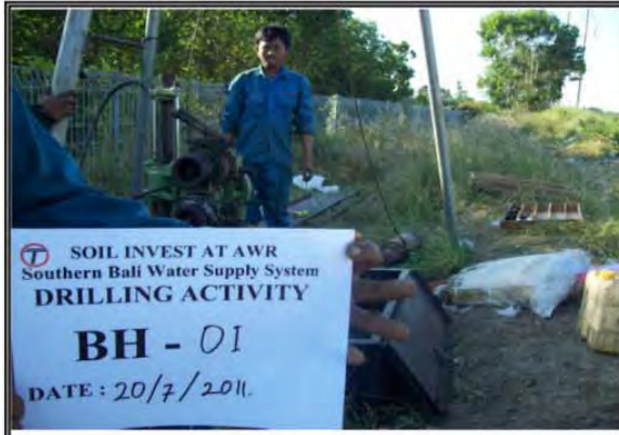
DRILLING AT BH-1
