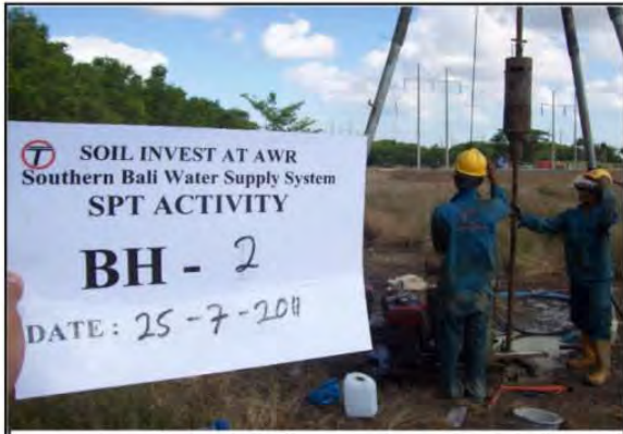
DRILLING AT BH-2
