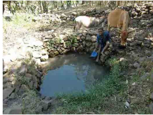
Livestock can access circled well easily. (Open well-1)
