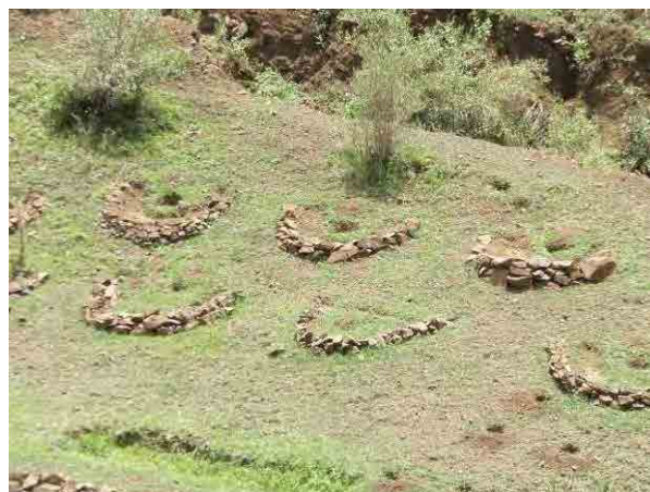
Water harvesting structures, such as half moon and micro-basin, can be used for tree plantation in the future.
