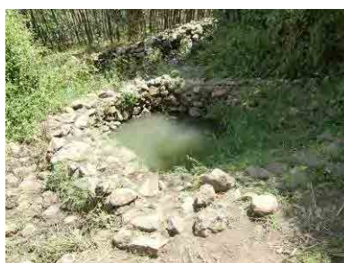
Open well-1 It is located beside the stream at 400m downstream from the target spring (Utilized for drinking)
