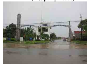
(6) Gate No. 2 (RC)
