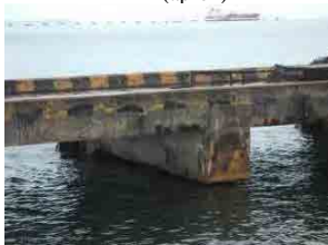
(14) Oil Jetty-3 (superstructure: side view)
