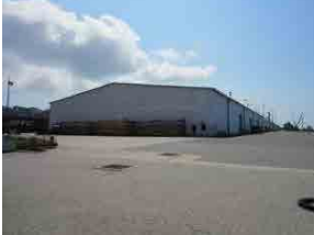
(5) Warehouse No. 5 (RC/Steel framed structure)
