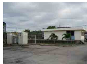
(3) Utility Building-1 (RC, pump house)
