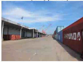
(5) Internal Road-2 (behind warehouse No.3)
