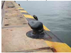
(8) Container Berth-4 (mooring bollard)
