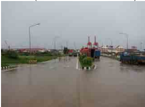
(7) Access Road (toward Gate No.3)
