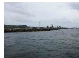
(9) North Breakwater (S)-4
