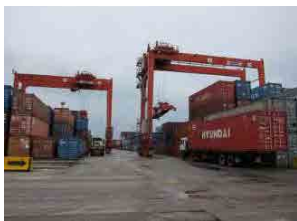
(1) Container Yard-1 (RTG foundations/ILB pavement)
