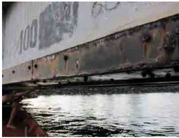
(32) Repaired P/C Beam (Access Brdg.) Type 6-1 (Steel plate encasement)
