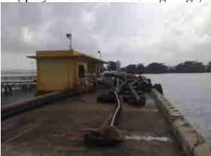
(13) Oil Jetty-2 (superstructure: upper view)
