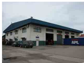
(2) Maintenance Workshop (RC/steel framed structure)
