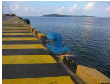
(5) Bollard (offshore side)
