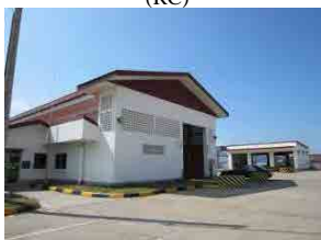
(8) X-ray Scanning Building (RC)
