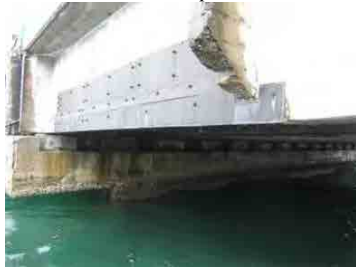
(19) Repaired P/C Beam (Main Pier) Type 6-2 (Steel plate encasement)
