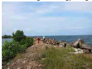
(1) North Breakwater (N)-1 (nearly original section portion)
