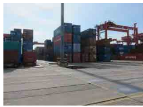
(2) Container Yard-2 (rainwater pooled)
