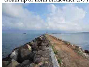
(8) North Breakwater (S)-3
