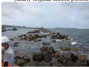
(4) North Breakwater (N)-4 (no stone materials exist)
