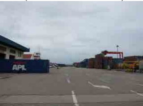
(8) CY Internal Road-1 (ILB pavement)
