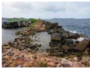
(2) North Breakwater (N)-2 (lacking stone fills portion)
