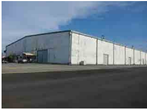
(1) Warehouse No. 1 (RC/Steel framed structure)
