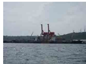
(៥១) Container Berth Basin-2
