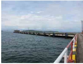
(1) Main Pier Overview
