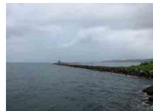
(6) North Breakwater (S)-1
