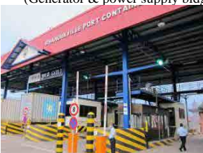
(7) Gate No. 3 (Steel Framed structure)
