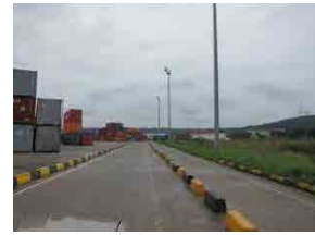
(3) West Port Road-3 (ILB pavement)
