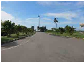
(1) West Port Road-1 (AC pavement)
