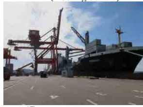
(5) Container Berth-1 (overview)
