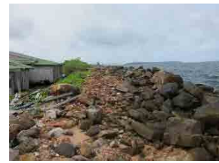
(3) North Breakwater (N)-3
