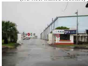
(5) Gate No. 1 (RC)
