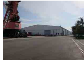
(3) Warehouse No. 3 (RC/Steel framed structure)
