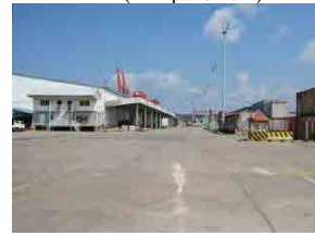
(6) Internal Road-3 (behind warehouses Nos. 4&5)
