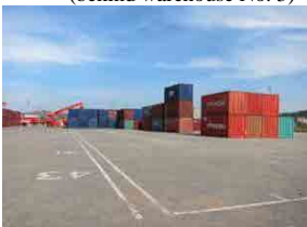
(4) Storage yard 2-1 (behind warehouses Nos. 4&5)
