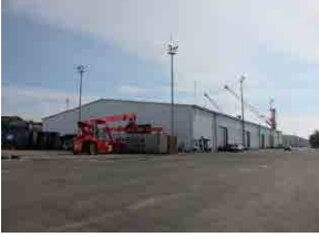
(4) Warehouse No. 4 (RC/Steel framed structure)
