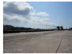
(3) Storage Yard 1-3 (behind warehouse No. 3)
