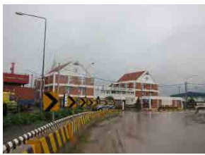
(1) Administration Building (RC, PAS office)
