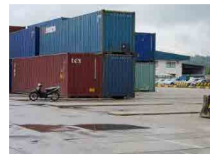
(3) Container Yard-3 (partially depressed)
