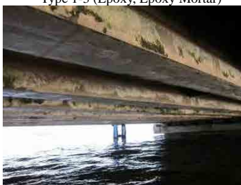
(26) Repaired P/C Beam (Main Pier) Type 1-3 (Epoxy, Epoxy Mortar)
