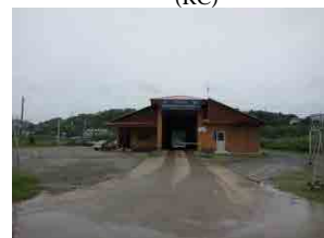
(9) Container Checking Building (RC, gamma-ray scanning system)
