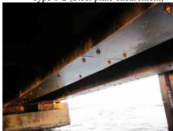
(22) Repaired P/C Beam (Main Pier) Type 6-2 (Steel plate encasement)
