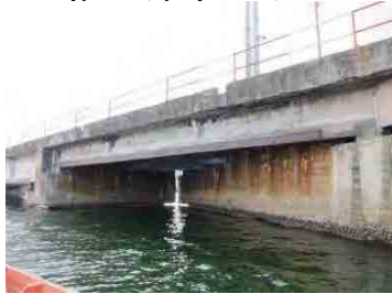
(37) Corner Junction Overview
