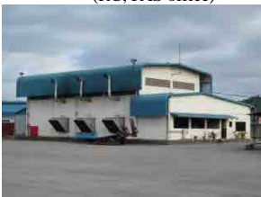
(4) Utility Building-2 (Generator & power supply bldg.)
