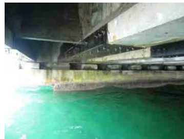
(18) Repaired P/C Beam (Main Pier) Type 6-1 (Steel plate encasement)
