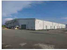
(2) Warehouse No. 2 (RC/Steel framed structure)
