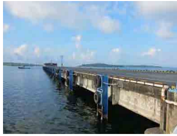
(2) Main Pier (inshore side)
