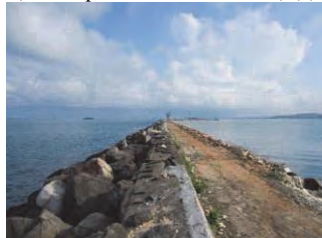
(8) North Breakwater (S)-3
