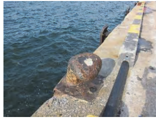
(2) New Quay-2 (mooring bollard)
