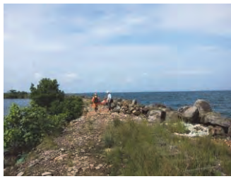
(1) North Breakwater (N)-1 (nearly original section portion)
