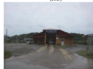
(9) Container Checking Building (RC, gamma-ray scanning system)
