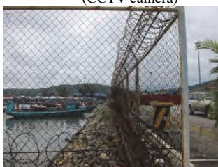
(17) Perimeter Fence-1 (Cyclone wire-type)
