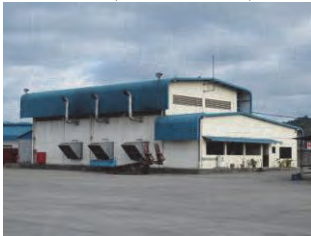
(4) Utility Building-2 (Generator & power supply bldg.)
