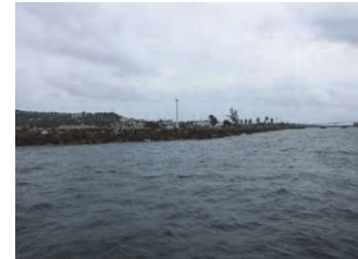
(9) North Breakwater (S)-4
