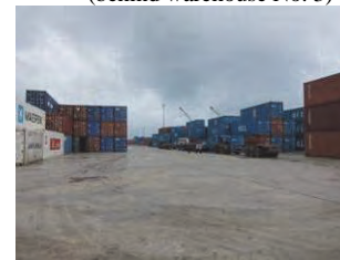
(6) Storage Yard 2-3 (behind warehouses Nos. 4&5)
