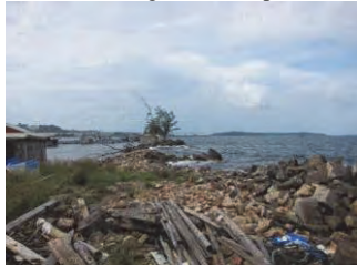
(5) North Breakwater (N)-5 (south tip of north breakwater (N) )
