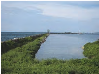
(7) North Breakwater (S)-2
