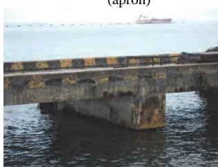
(14) Oil Jetty-3 (superstructure: side view)
