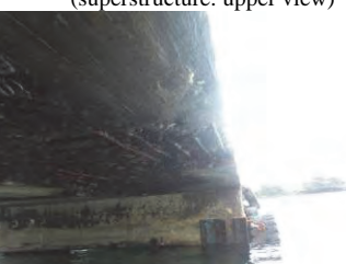
(16) Oil Jetty-5 (superstructure: underneath view)
