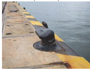
(8) Container Berth-4 (mooring bollard)
