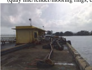
(13) Oil Jetty-2 (superstructure: upper view)
