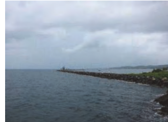
(6) North Breakwater (S)-1
