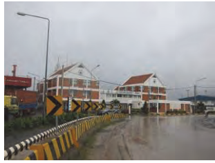
(1) Administration Building (RC, PAS office)
