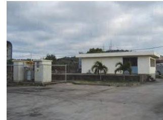
(3) Utility Building-1 (RC, pump house)
