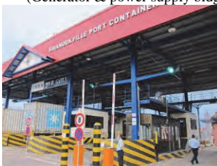
(7) Gate No. 3 (Steel framed structure)
