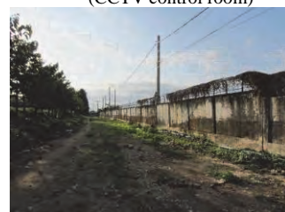
(18) Perimeter Fence-2 (Concrete wall type)
