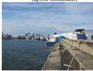
(10) Tugboat Quay-2 (quay line/fender/mooring rings, etc.)
