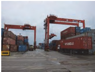
(1) Container Yard-1 (RTG foundations/ILB pavement)
