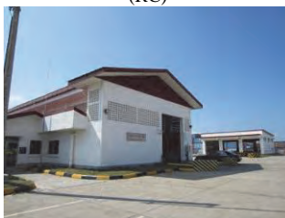
(8) X-ray Scanning Building (RC)
