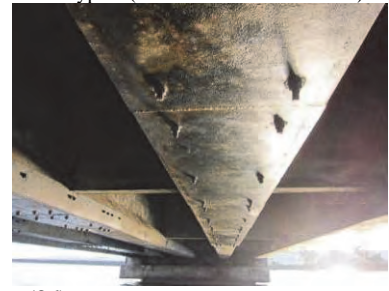
(36) Repaired P/C Beam (Access Brdg.) Type 6-1 (Steel Plate Encasement)
