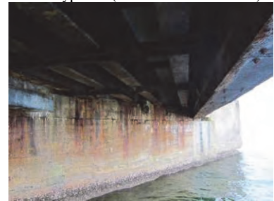
(39) Repaired P/C Beam (Cnr. Junction) Replaced by H-shaped Steel Beam
