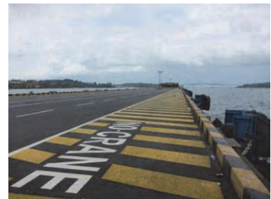
(12) Apron (offshore side) Restriction Markings
