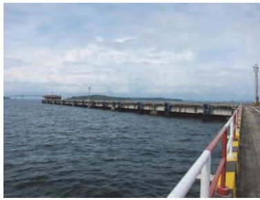
(1) Main Pier Overview
