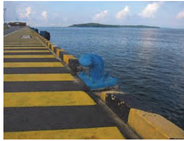
(5) Bollard (offshore side)
