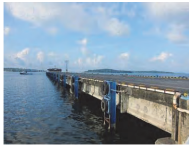
(2) Main Pier (inshore side)
