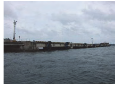
(3) Main Pier (offshore side)
