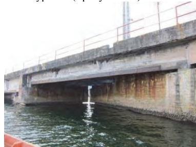
(37) Corner Junction Overview
