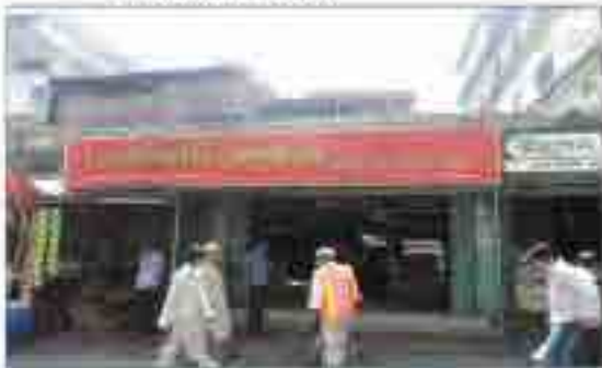
Photo of Structure
