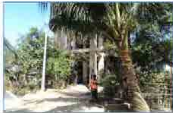
Gate Valve (Over Head Tank Location)
