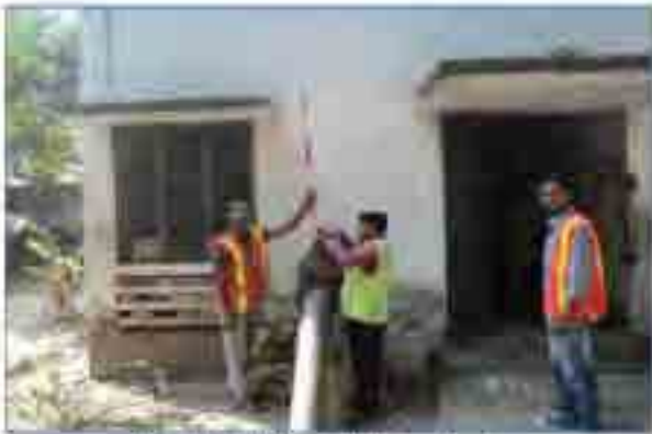
Gate Valve (Deep Well Location)
