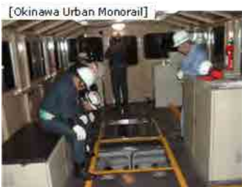
G. Inside Mobile work-shop(Visual inspection of track)
