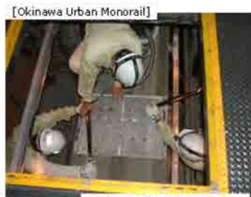
H. Inspection of track bolts
