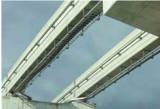
Figure 6-7 Contact Wire and Cable Tray
