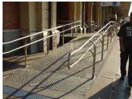
Slope for wheel chair in metro station
