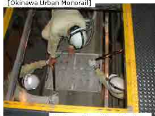
H. Inspection of track bolts
