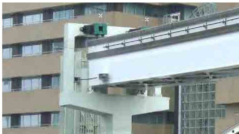
Figure 5-41 Photo of the stoppers, End of TAMA MONORAIL
