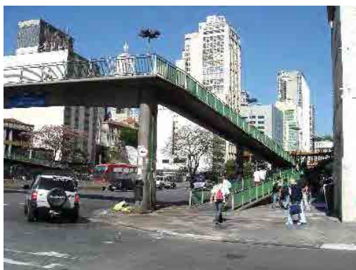
Pedestrian bridge with slope Source: JICA Study team
