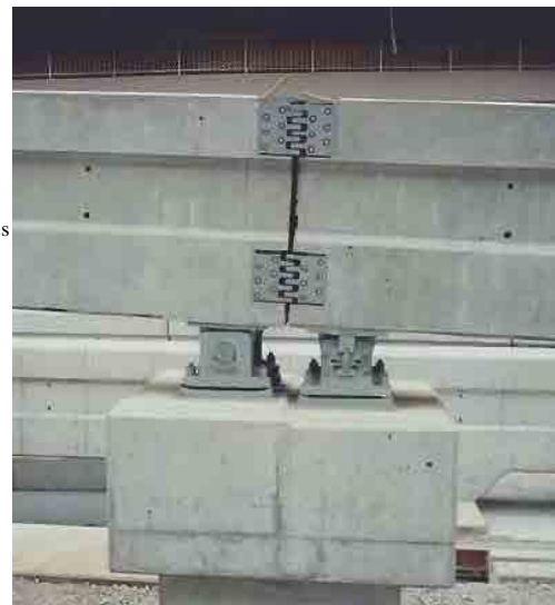
Figure 5-40 Bearings and Expansion Joints (Example)
