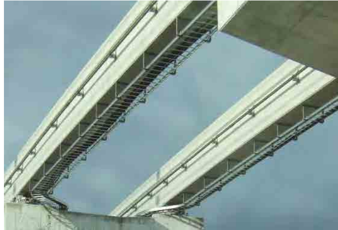
Figure 1-17 Cable tray and contact line
