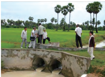
Turnout/ Check structure constructed by TSC3
