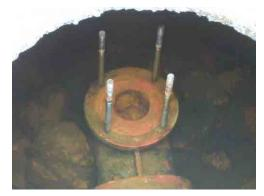
Figure 9.5.2 Damaged air valve
