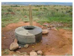
Figure 9.5.1 Signs of theft of water on air valve chamber
