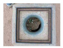
Figure 4.3.2 Buried Valve Head
