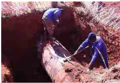
Visual inspection (Dry area)
