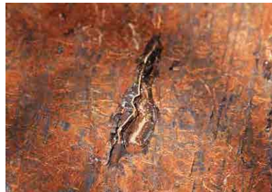
Coating damaged (※3)
