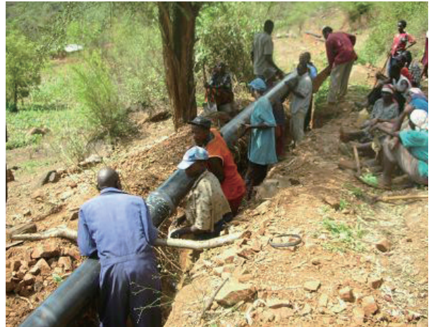
Pipe installation by farmers in Kiambindu
