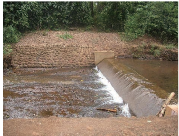
Intake weir constructed by the Project in Kisioki
