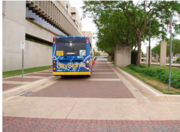
Figure 6.4.2 Brisbane example off paving a BRT only carriageway
