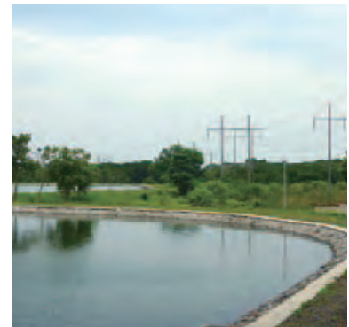
Stabilization pond at the wastewater treatment plant
