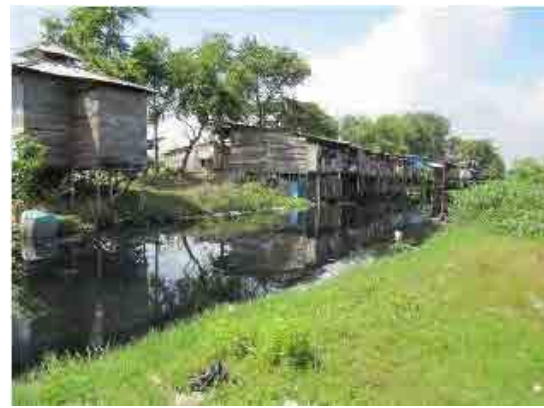
Figure B3-27 Houses with Bad Air Circulation
