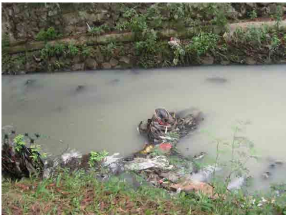
Drainage is contaminated by sewage and solid wastes in Jakarta.
