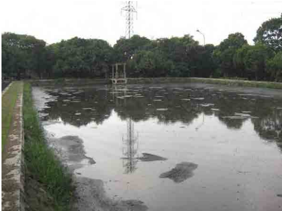
Existing Duri Kosambi sludge treatment plant.
