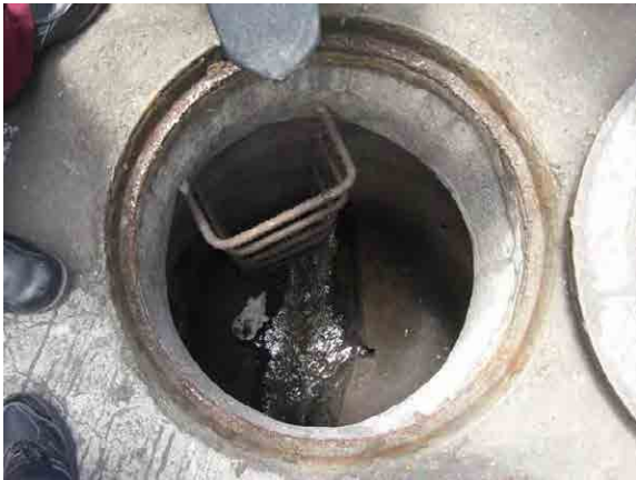
Inside of the existing manhole.
