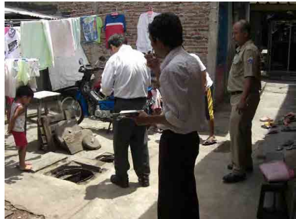
Condition of septic tank in the slum area.
