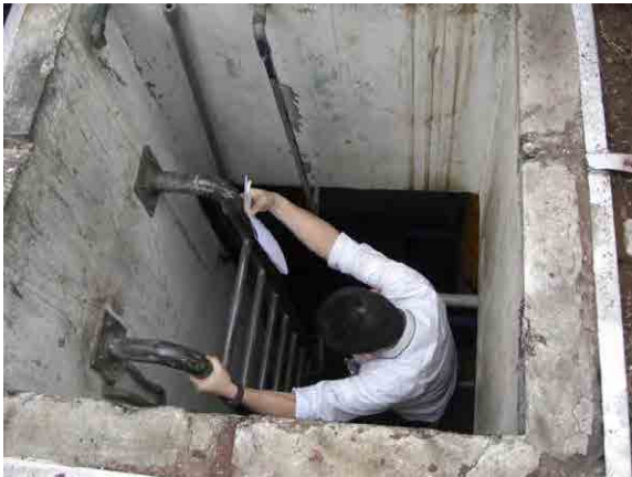
Condition of the individual treatment plant.
