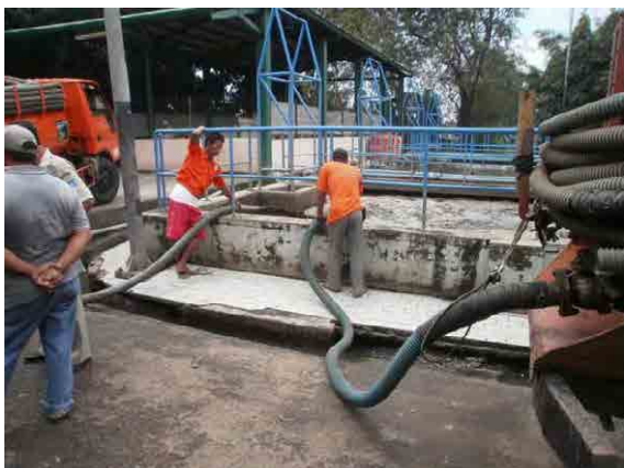
On-site sludge is discharged into receiving tank at the existing sludge treatment plant.
