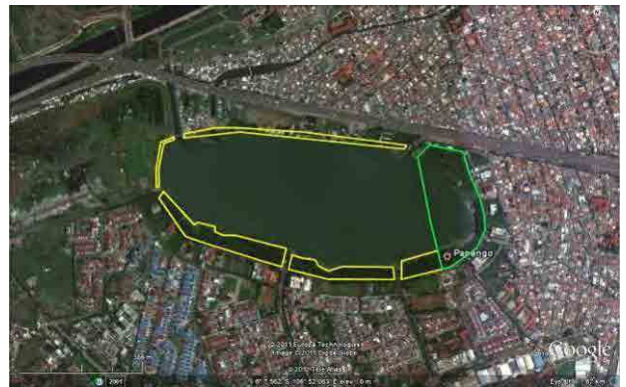
Site No. 5) Zone 5 WWTP (City Forest North Sunter Pond)
