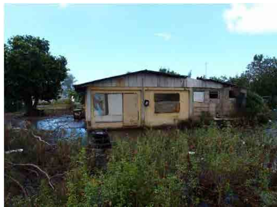
Abandoned house due to drainage, in Nuku'alofa, Tonga (Feb, 2012)
