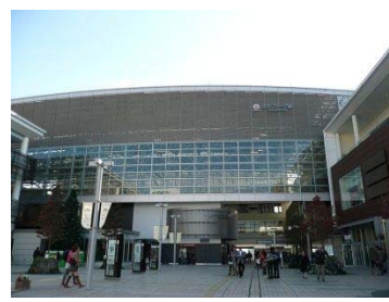
Station Yard in Present 2/
