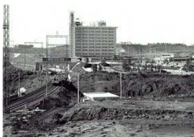
Under construction in late 1960s 1/
