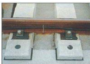
Photo 2.3.3.4-1 Direct Fixation Track
