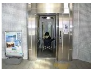
Elevator for Universal Access
