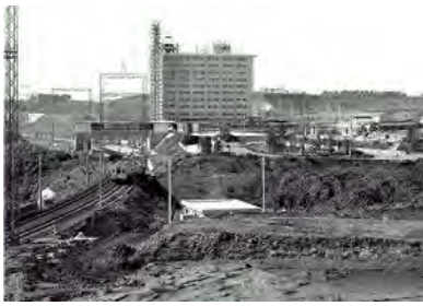
Under construction in late 1960s 1/
