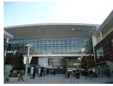
Station Yard in Present 2/
