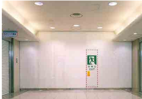
Figure 5-9 Fire Protection Compartment (Screen Type) with Door
