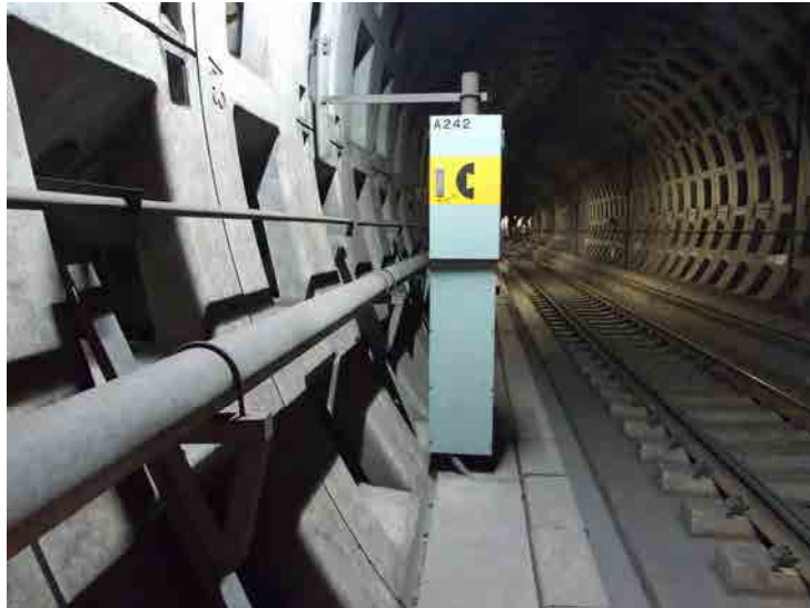
Figure 5-5 Telecommunication System in Tunnel
