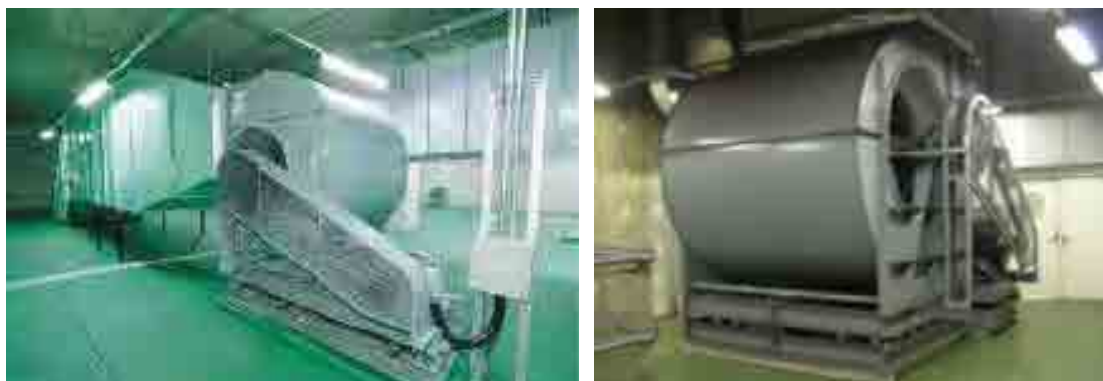
Figure 4-3 Exhaust of smoke in tunnel
