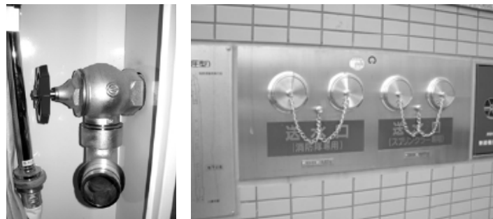
Figure 5-12 Example of Hydrant for Water Outlet in Station (Left) and Siamese Connection for Water Supply on Ground Level (Right)
