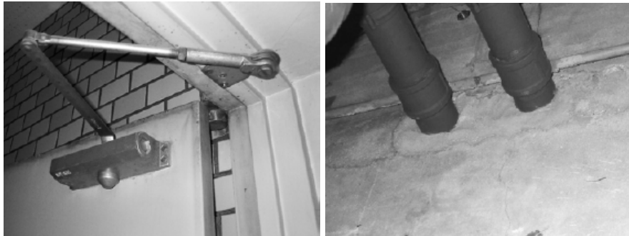
Figure 2-2 Automatic Door Closer for Compartment Room and Void filled by Non Combustible Material
