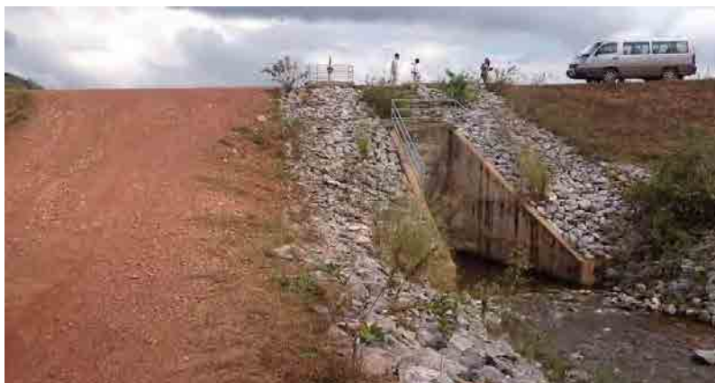
Existing water gate at Tak Krola dam
