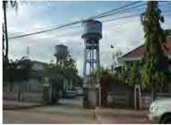
Elevated tanks in Kampot WTP
