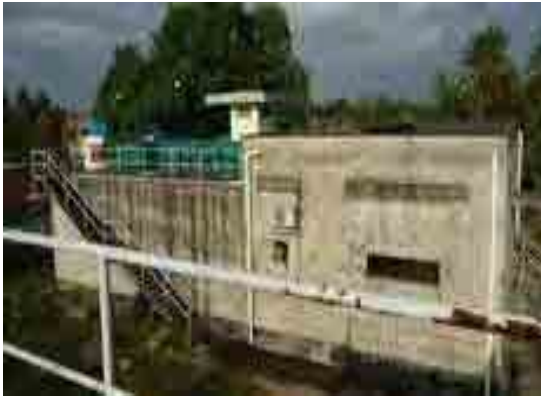
Kampot existing Water Treatment Plant (WTP)
