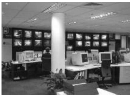
Control Centre Brisbane
