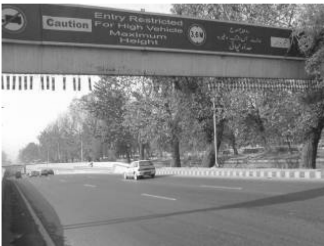
Figure 3.4.12 Low Height Underpass with 3.6m Vertical Clearance
