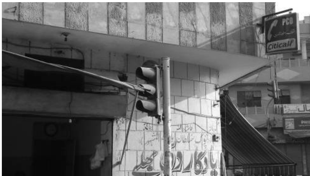
Figure 3.4.20 Traffic Signal Covered by Shop Shade
