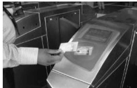
Smart card ticketing at turnstiles records each trip at allows free transfer across the network
