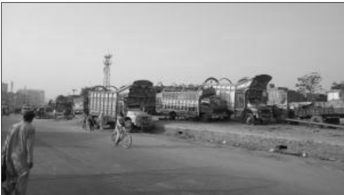
Figure 8.5.7 Condition of Existing Truck Stand/ Terminal at Sabzazar
